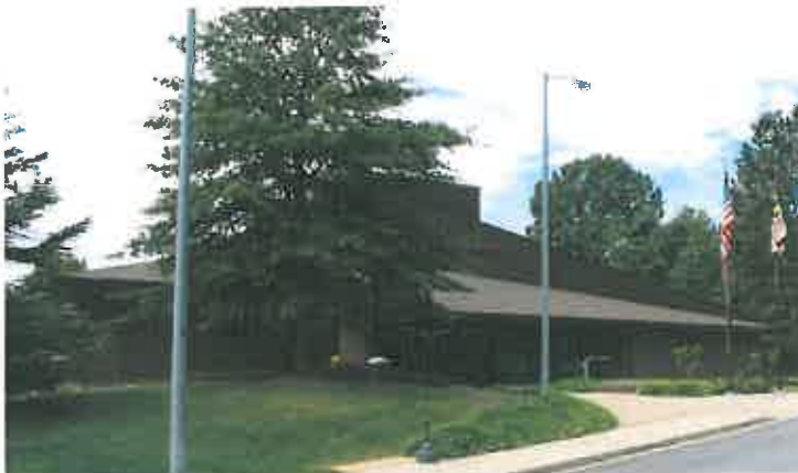
Maryland Welcome Center, Crain Memorial Highway at the Potomac River crossing, Charles County
