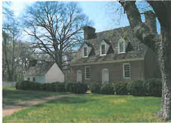
Smallwood's Retreat House, Smallwood State Park, Charles County
